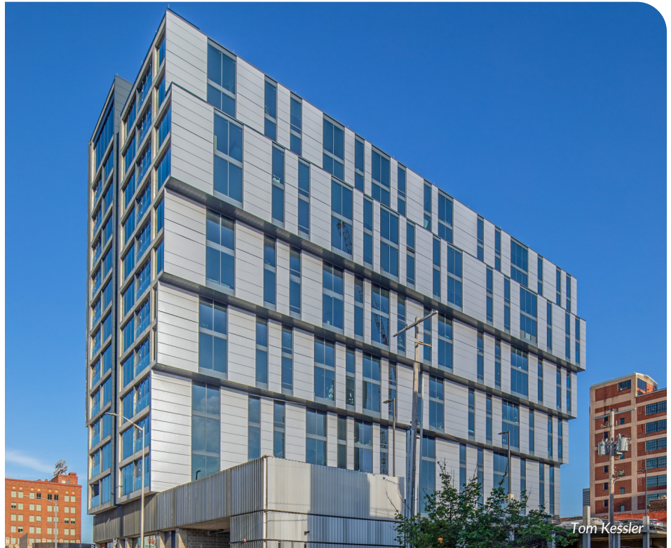
To blend with Crossroads' historic brick buildings and exposed concrete structures, Burns & McDonnell specified dark aluminum framing, insulated metal panels, exposed concrete and prefinished metal trim together with Solarban® high-performance solar control low-e glass.
